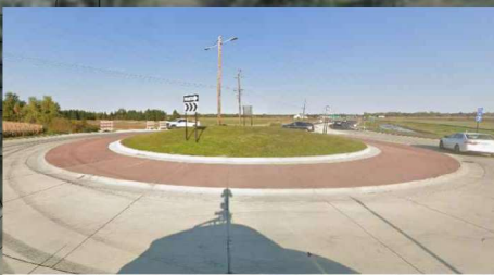
STREET VIEW FROM SOUTHWEST
