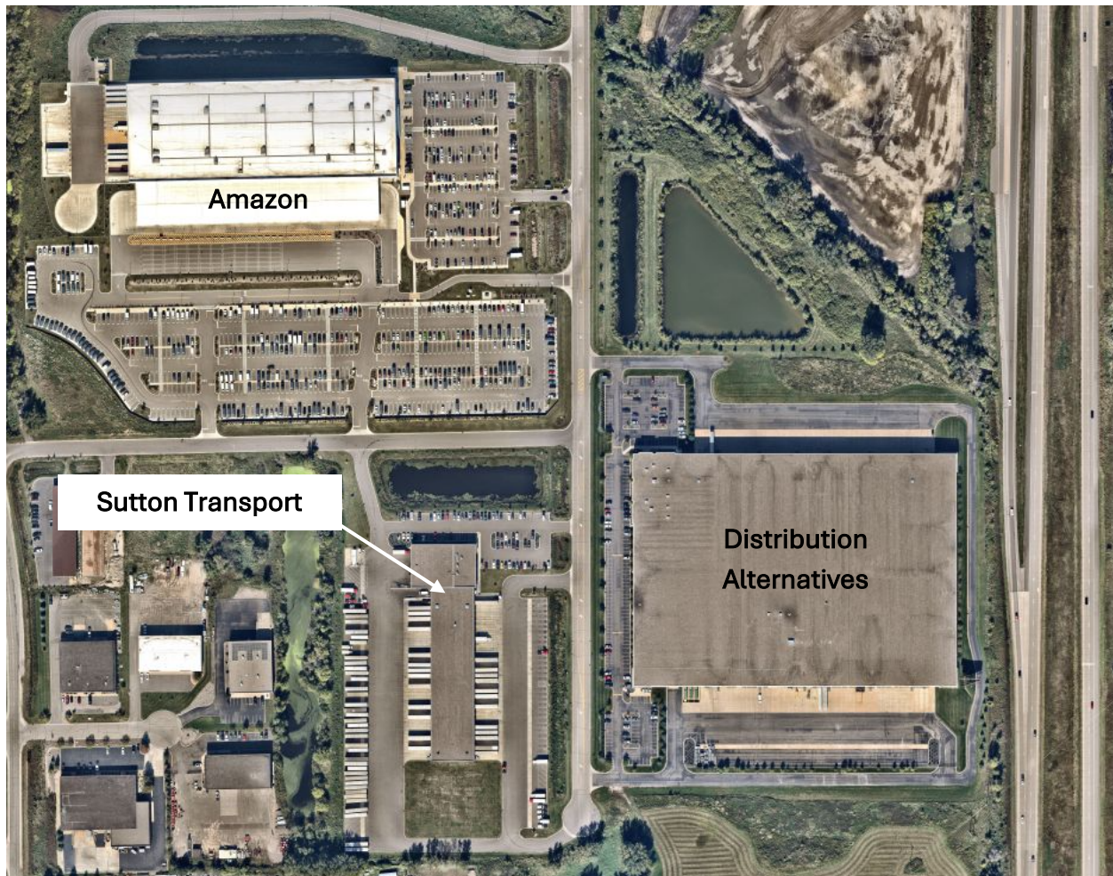
Figure 1 Distribution Alternatives, 6870 21st Ave S, Lino Lakes, MN 55038
