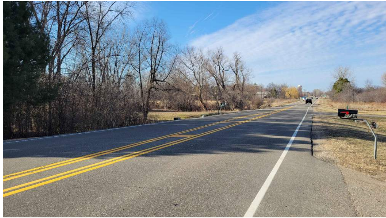
PHOTO 4 VIEW LOOKING NORTH ALONG 20TH AVE S.
